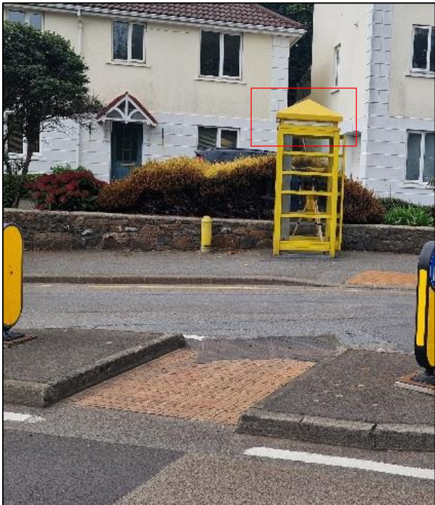
Trinity Hill Kiosk (bottom of Trinity Road) - 5.02% of ICNIRP guidelines
